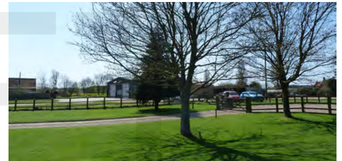
The barn at Morston Hall Farm is atypical in terms of scale and materials but is set back from the road and screened by trees and fences
