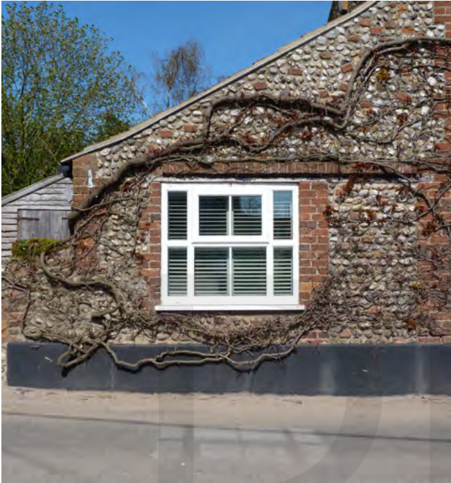
uPVC window on The Street. Its white colour contrasts starkly with the brick and flint work, while the top-hung casement is atypical of the Conservation Area
